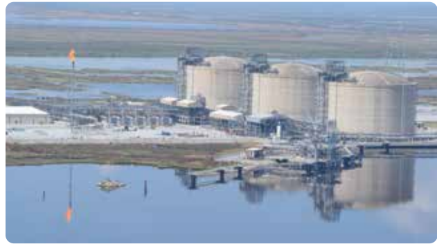
THE CAMERON LNG FACILITY FLARING, WHERE METHANE GAS IS BURNED AND POLLUTANTS ARE RELEASED. SEPTEMBER 6, 2020. PHOTO: © HEALTHY GULF, COURTESY SOUTHWINGS
